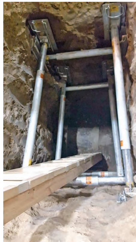
The excavations were deeper than 5 feet, requiring an OSHA approved trench protection system. To shore the pits, the contractor employed four, single-cylinder hydraulic "spot-shores;" two running in each direction. When activated, the hydraulic pressure from the cylinders prevents the trench walls from collapsing.
