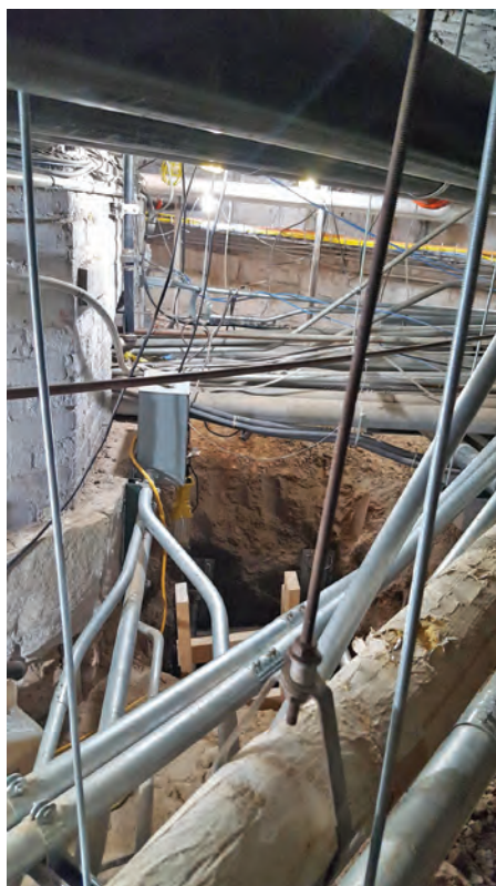
Renovation of Michigan's historic Capitol Building's 150-years old plumbing required hand-digging 8-foot deep "excavations" in a five-foot crawl space under the building's historic rotunda.
