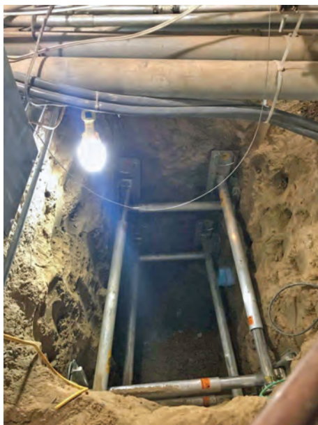
The alignment hole for the pipe lining of a section of the building's original 1872-constructed sanitation pipe was partially dug under a conduit two feet off the floor.
