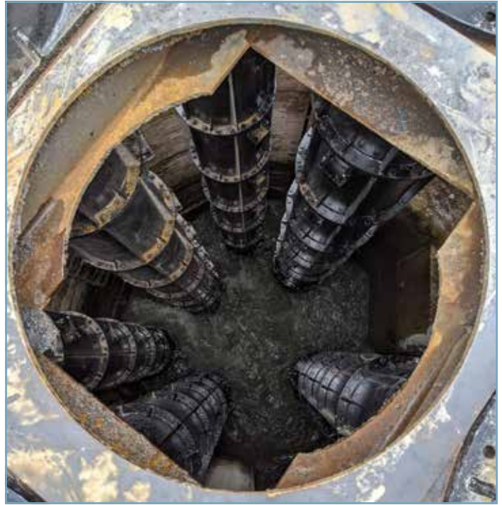
View from the last pump base plate porthole before the 7th and final pump was installed into the bypass pumping structure (Gate House Shaft).
