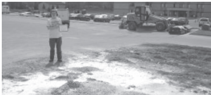
Concrete truck washout should only be discharged in designated areas.
