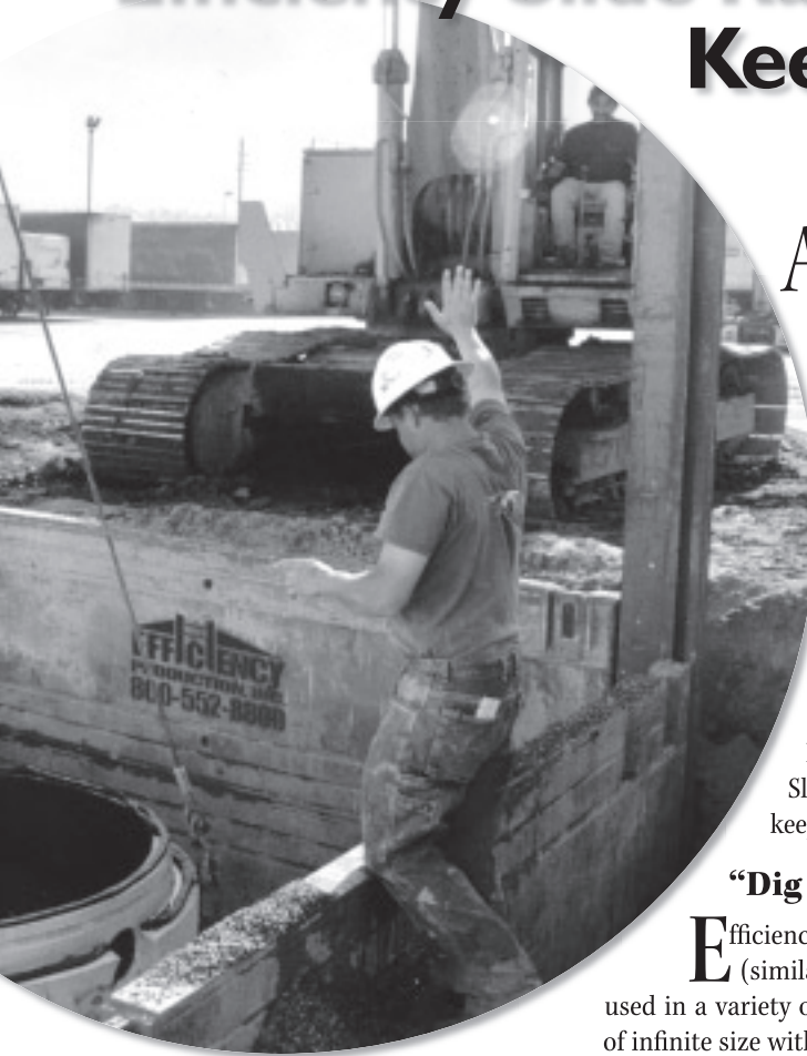
Joe Raica Excavating was contracted to install a new pre-cast lift station in Howell.
