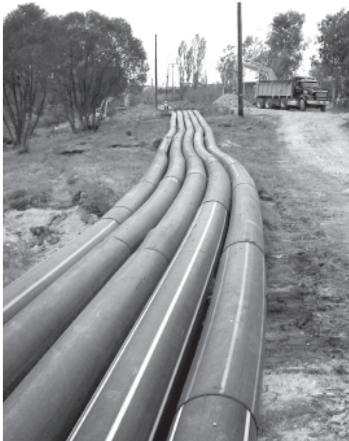
Ontario Creek Bypass Project: 60,000 GPM over two miles of fused 18-inch discharge pipe.
