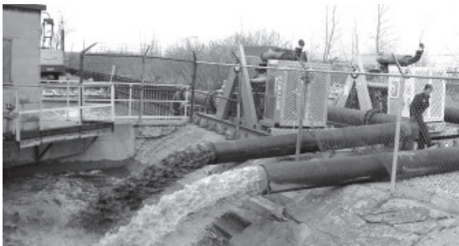
18 inch discharge pipes running full.
