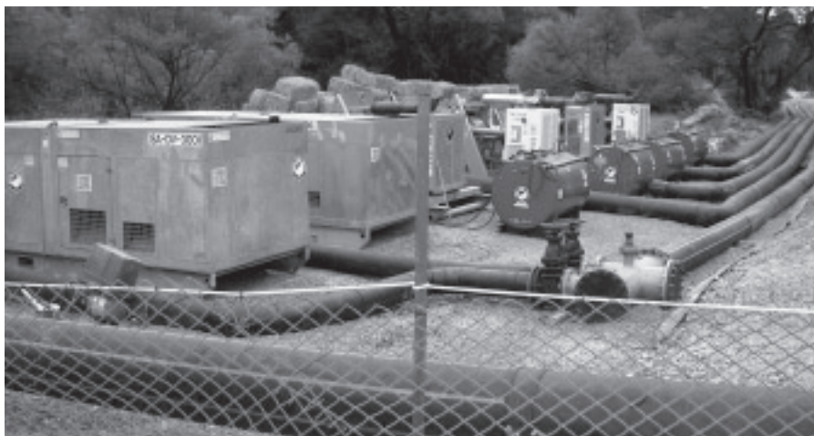
DV300I 12' High Flow (6,900 GPM) Auto Prime Trash Pump. The unit is housed in a sound attenuated enclosure to allow for quiet running in noise sensitive areas.
