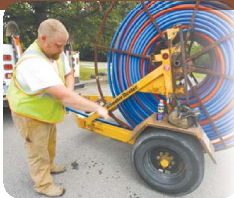
Bill Winter is getting ready to attach the heavy-duty innerduct to the end of the boring head. The boring rig will then pull it back through the hole with locating wire attached. Fiber optic is installed in innerduct and heat spliced in hand-holes where necessary.
