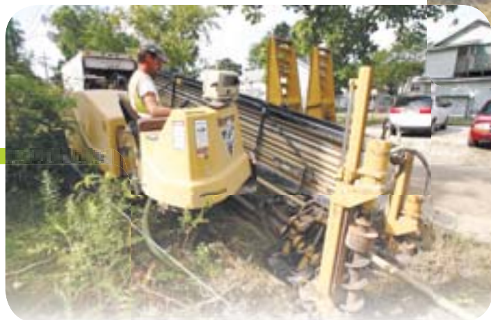
Steve Voshell operating the boring machine as its auto-loader of pipe slides into position and auto-threads next section to push on and extend boring length.
