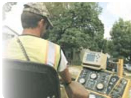
Steve Voshell operates the boring machine checking direction and depth of boring head from electronics.
