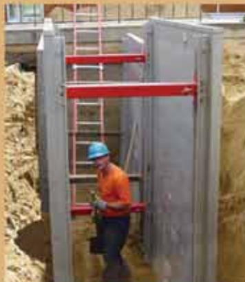
Aluminum Trench Shields
