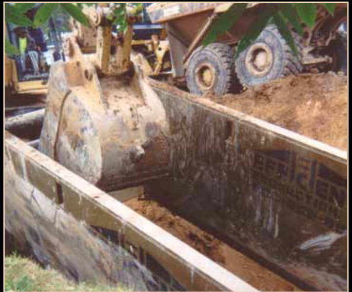
Steel Trench Shields
