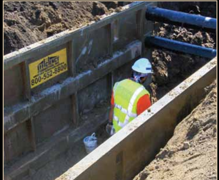
Steel Trench Shields
