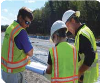
Joe Goodall of Dan's Excavating (left) and Tia Klein of FTCH (middle) show the site plans to State Rep. Dan Lauwers (right).
