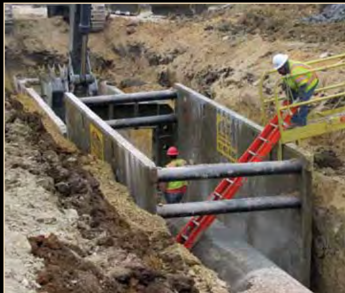
Steel Trench Shields
