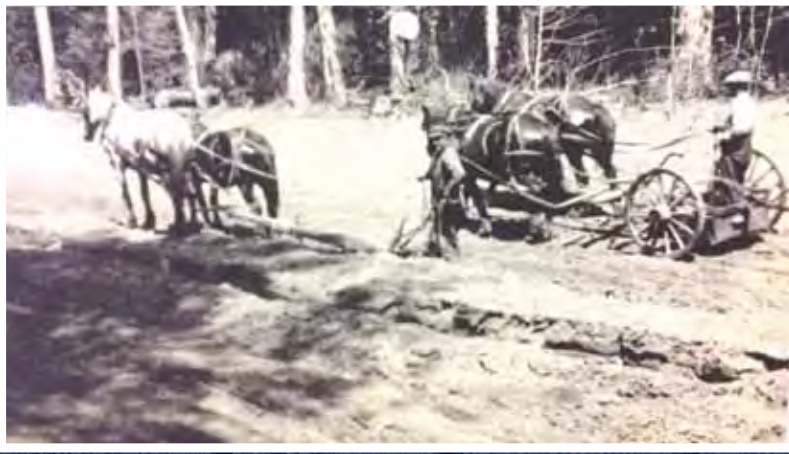
Plowing and wheeling from cut at M-35 in 1926.
