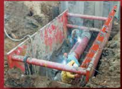
STEEL TRENCH SHIELDS
