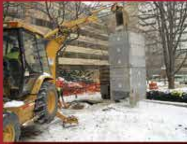
ALUMINUM TRENCH SHIELDS
