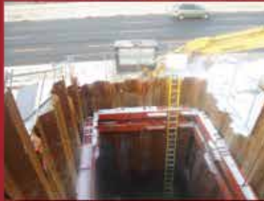
PRO-BRACE HYDRAULIC FRAME
