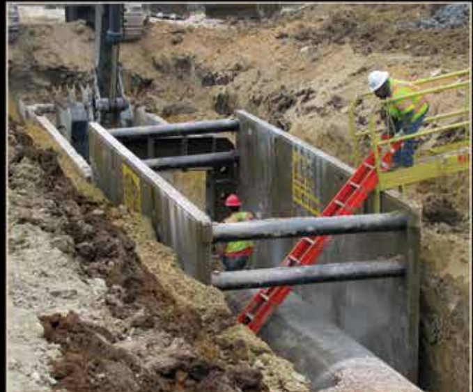
Steel Trench Shields
