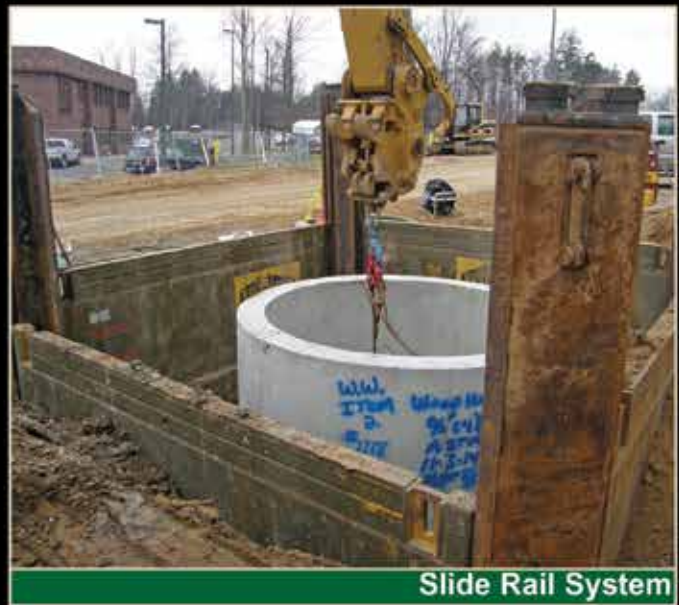
Steel Trench Shields
