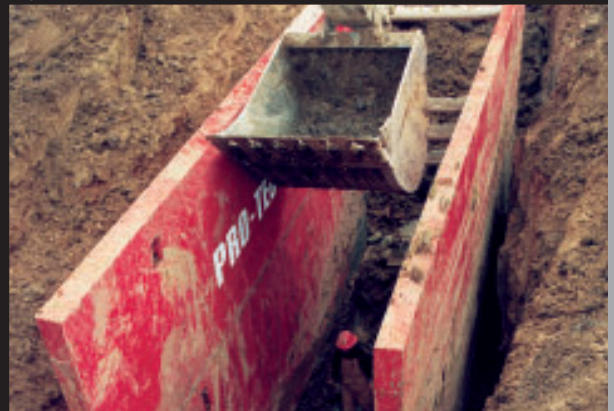
Steel Trench Shields
