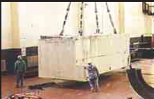
The crane removes a multi-ton section from inside the plant to be cut into smaller pieces.
