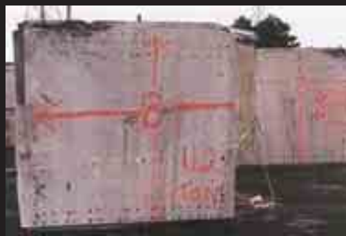
112-ton concrete section removed from plant.
