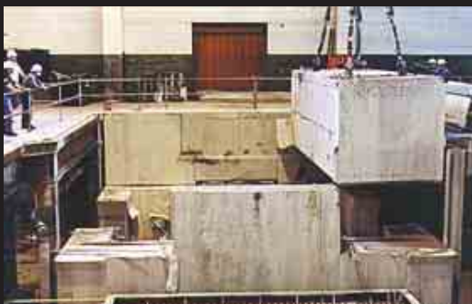
The crane removes a multi-ton section from inside the plant to be cut into smaller pieces.
