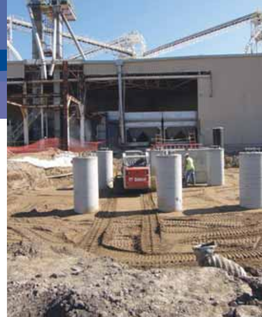
The completed pour-in-place structure will contain an auger "alley pit" for grain movement within the elevator facility.
