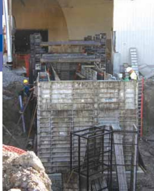
The excavation for the alley pit vault was unusual in that though relatively shallow—16 feet deep—the long trench needed to be dug two-thirds outside and one-third inside an existing building.
