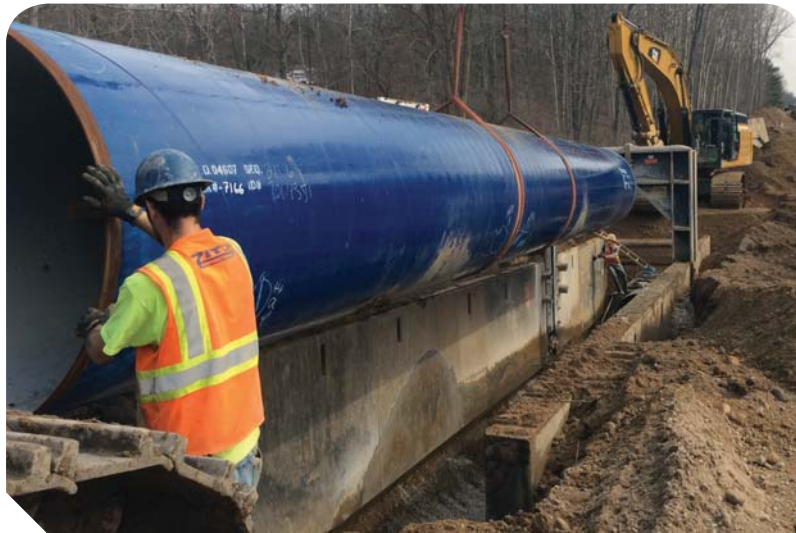
Zito is installing 50 foot long sections of 60 inch diameter steel spiral-weld pipe 13 miles along the main transmission line of the KWA pipeline project. The boundaries of the new water supply will encompass over 2,400 square miles and over a half million people.
