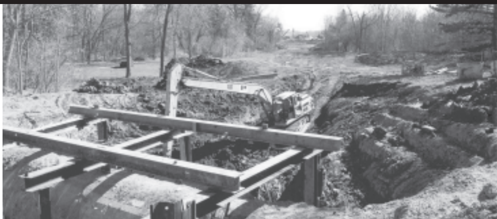
G2 Consulting Group recently engineered the sinking of a 20-million-pound concrete pipe 95 feet below ground. This will help prevent sewage overflows into the Rouge River in Dearborn, Mich.
