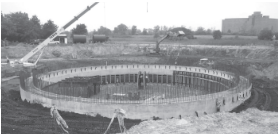
G2 Consulting Group recently engineered the sinking of a 20-million-pound concrete pipe 95 feet below ground. This will help prevent sewage overflows into the Rouge River in Dearborn, Mich.
