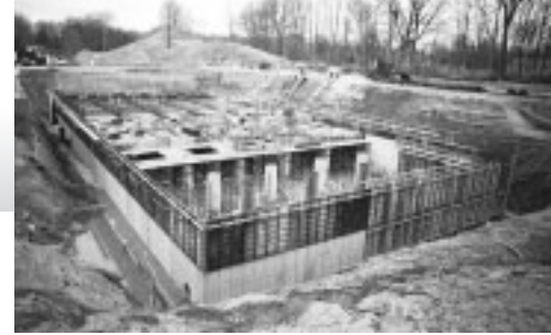
Storing backfill material on an adjacent private property was a cost-effective solution for the basin's tight construction area.
