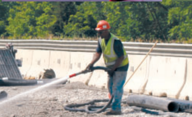
Removing false decking from a new superstructure in Grand Rapids
