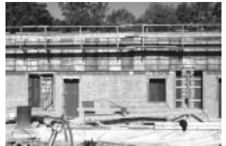
Tinted concrete and a formliner were used to create a stonewall look for the control building.
