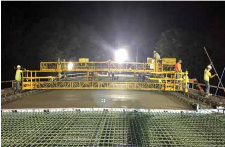
▶ Bridge deck pour on Cheney Avenue over I-96 in Kent County.
