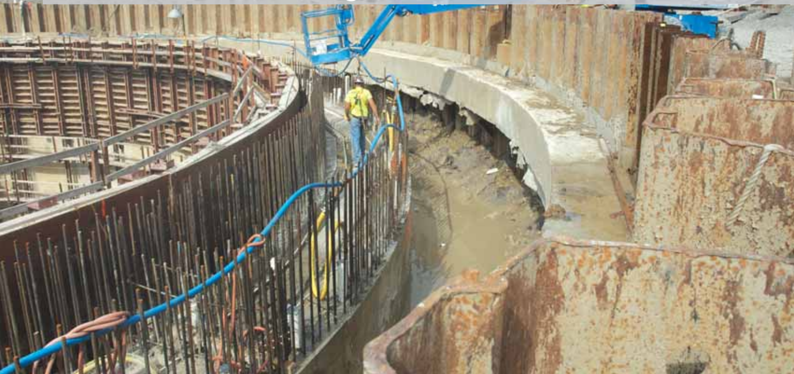
Above ground view of caisson with partial forms.
