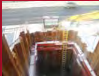
PRO-BRACE HYDRAULIC FRAME
