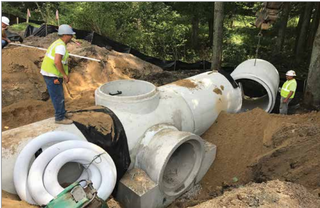
C&D Hughes installing 60' RCP to replace 16-year-old failed HDPE pipe in Fowlerville, Mich.
