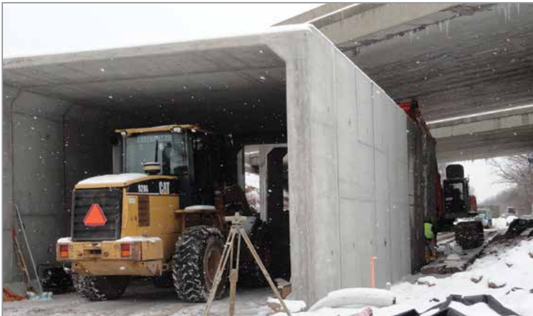
Anlaan Corporation installing the Portland Pedestrian Tunnel under I-96.
