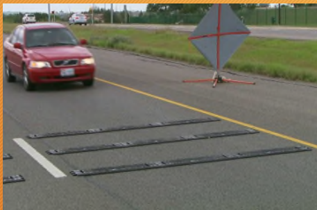
Temporary Rumble Strips
