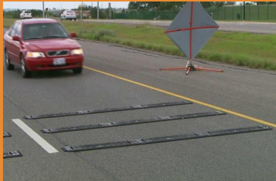
Temporary Rumble Strips
