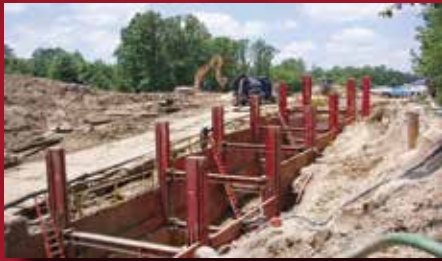
SLIDE RAIL SHORING
