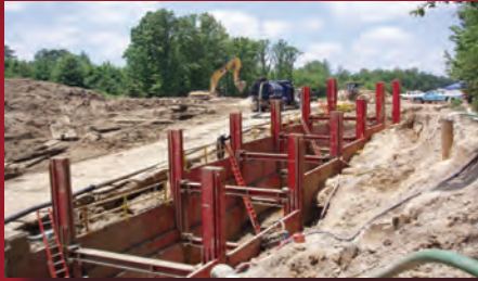
SLIDE RAIL SHORING
