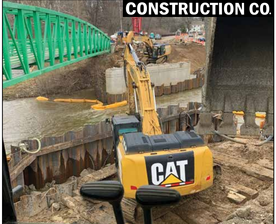
The Okemos Road Bridge Project
