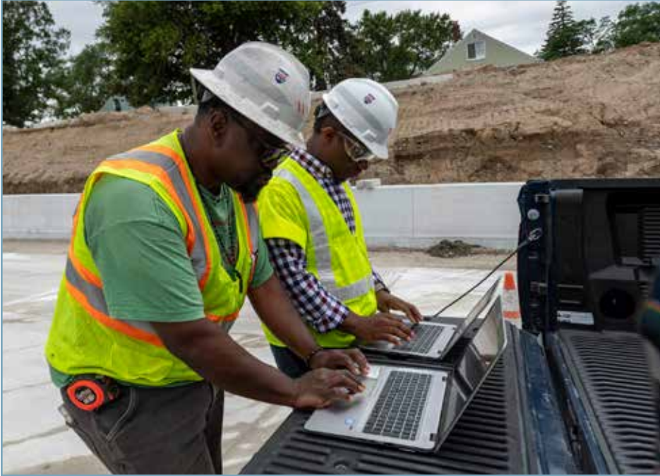
Team members access digital plans while on site at Segment 3 of the MDOT I-75 modernization project in the department's Metro Region in June 2021. (MDOT photo)
