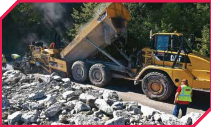
CAT 725 off road truck feeding CAT paver on M-185, Mackinac Island
