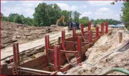
SLIDE RAIL SHORING
