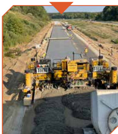
Toebe Construction, LLC, uses a Gomaco GHP 2800 paver on the Interstate 69 project in Lapeer County. Photos courtesy of Toebe Construction, LLC.
