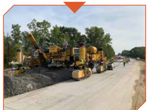
Toebe Construction, LLC, uses a Gomaco GHP 2800 paver on the Interstate 69 project in Lapeer County. Photos courtesy of Toebe Construction, LLC.
