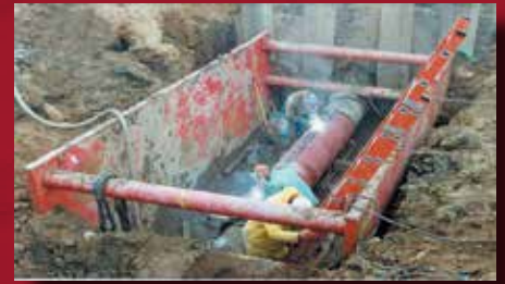
STEEL TRENCH SHIELDS
