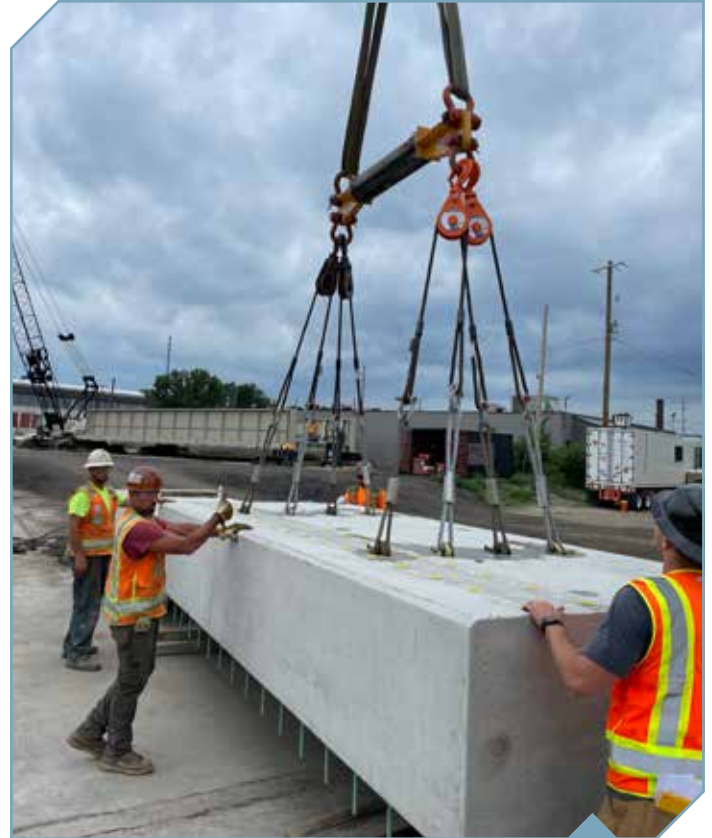
The precast abutment top is erected at the bridge over Jackson Street. Photo Courtesy of Anlaan Corporation
