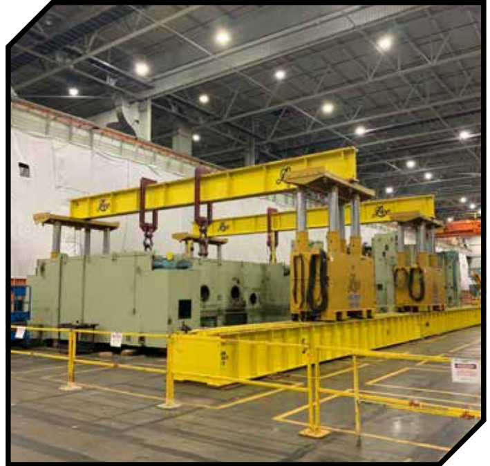
600,000 lb. Transfer Press Crown Removal.
