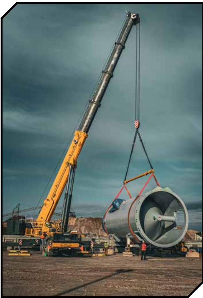
Setting (2) massive granulation basins onto a barge.
