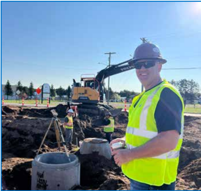
Greg Brooks visiting M & M's Jobsite in Northern Michigan.
