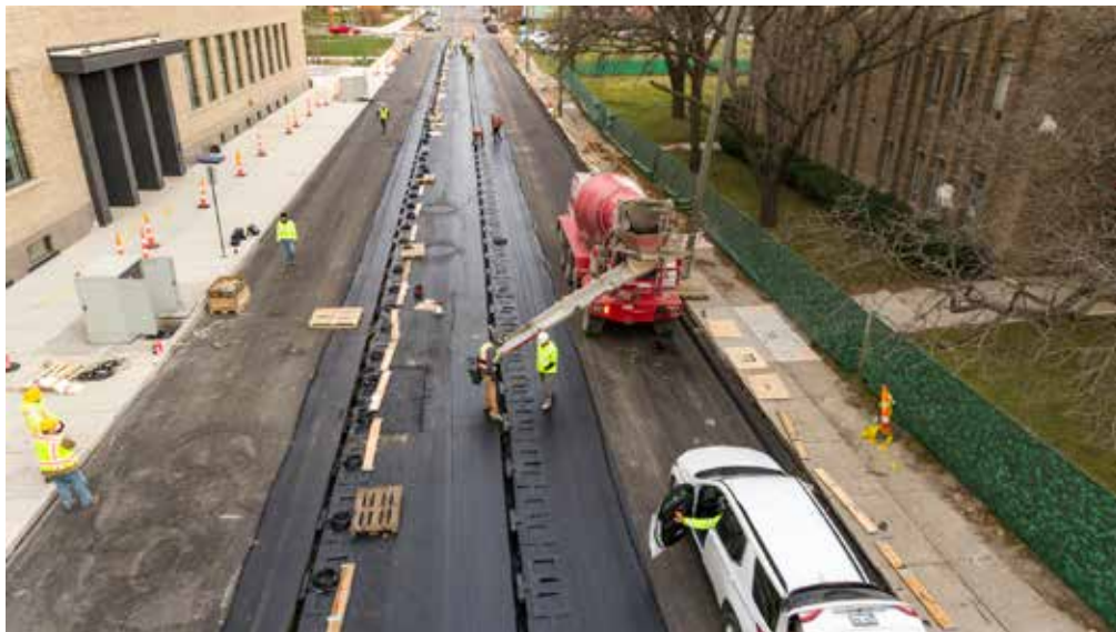
Concrete is poured on the 14th Street wireless charging project. Photos courtesy of MDOT.
