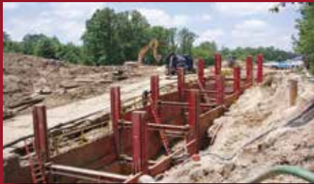
SLIDE RAIL SHORING
