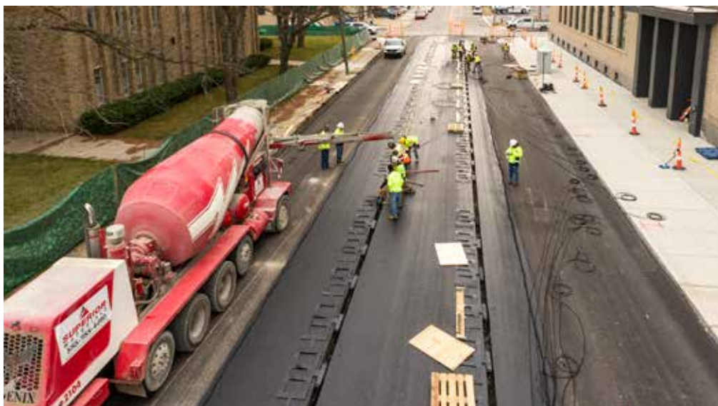
Concrete is poured on the 14th Street wireless charging project. Photos courtesy of MDOT.
