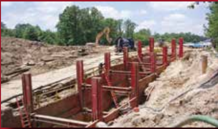
SLIDE RAIL SHORING
