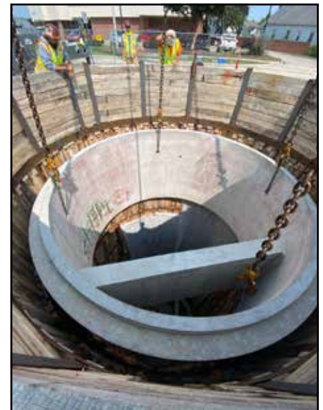
168" Shafts for the I-75 Modernization Project Segment 3, which NCP is working on this year in Oakland County.
