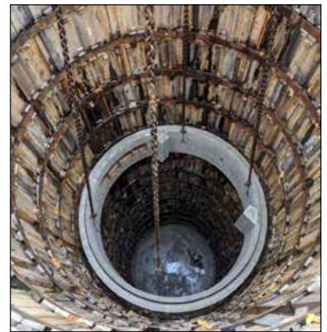
168" Shafts for the I-75 Modernization Project Segment 3, which NCP is working on this year in Oakland County.
