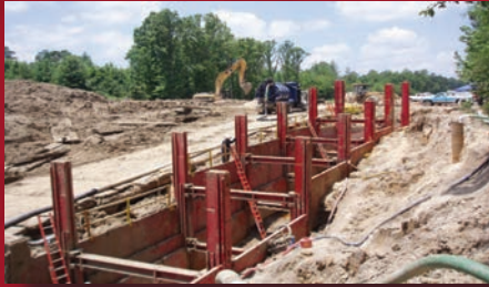
SLIDE RAIL SHORING
