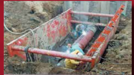
STEEL TRENCH SHIELDS
