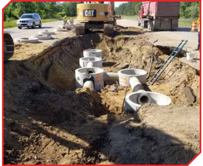
Kalin installing storm sewer in the median of US 127.
