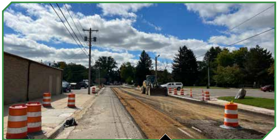
Wellesly Storm Water Repair, Lansing, MI.
