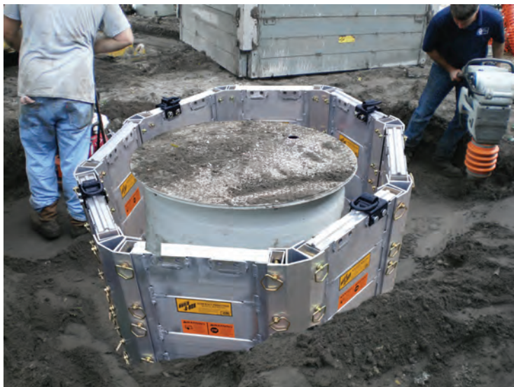
Efficiency Production's new octagon-configured trench shield.
