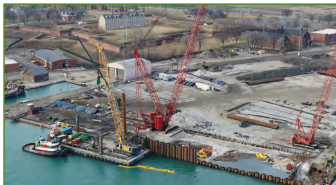
January 2021: Left – undisturbed zone with the new seawall installation complete.
