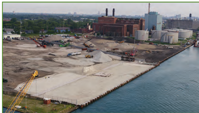
August 2021: Revere Dock site after construction, showing new seawall and Great Lakes Water Authority outfall structure in place and operational.
