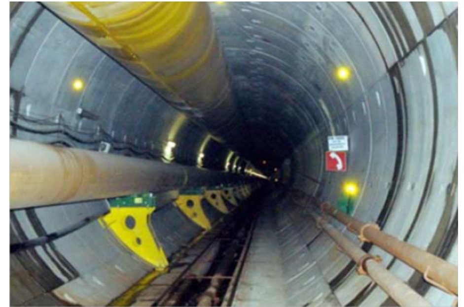
Gastau tunnel (Brazil): 17.5 ft internal diameter
