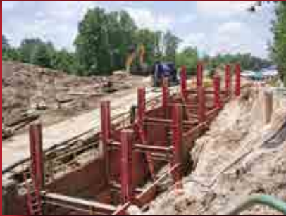
SLIDE RAIL SHORING
