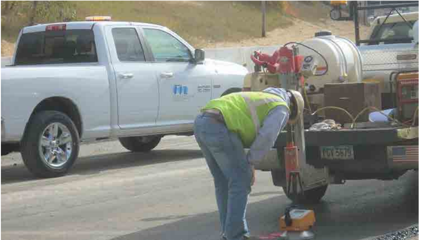
TTL's engineering technician performing quality control testing and inspection.
