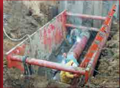
STEEL TRENCH SHIELDS
