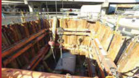
PRO-BRACE HYDRAULIC FRAME
