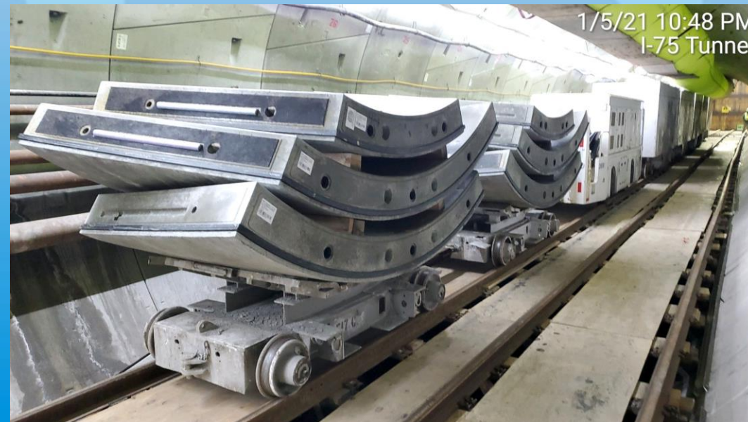
Inside the Tunnel – Precast Concrete Segments Waiting Delivery to the Tunnel “Heading”
