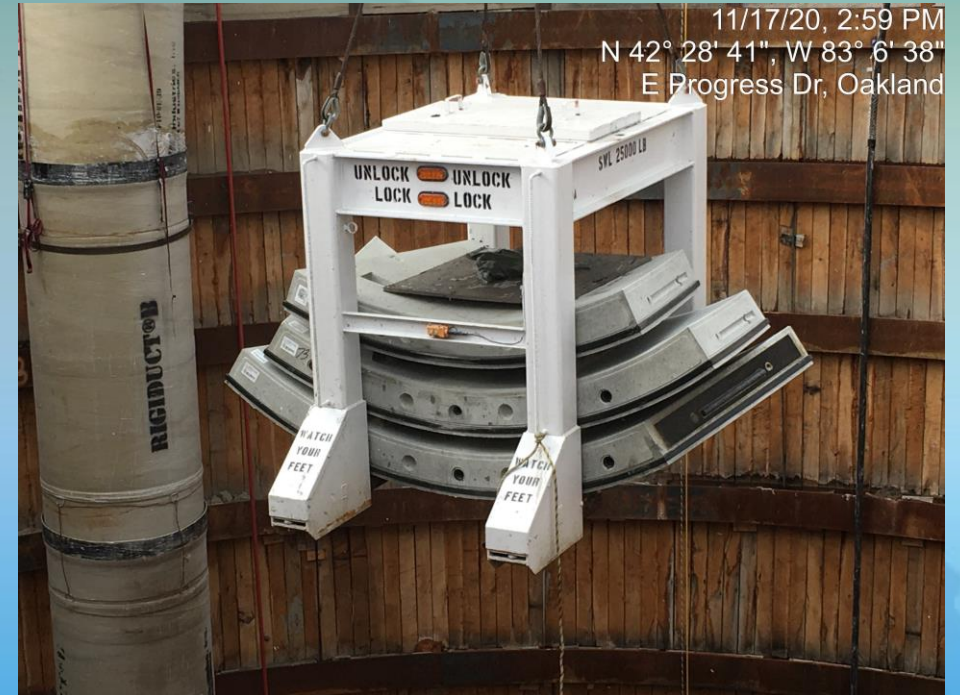
Precast Tunnel Segments Being Lowered to Bottom of the 696 Shaft
