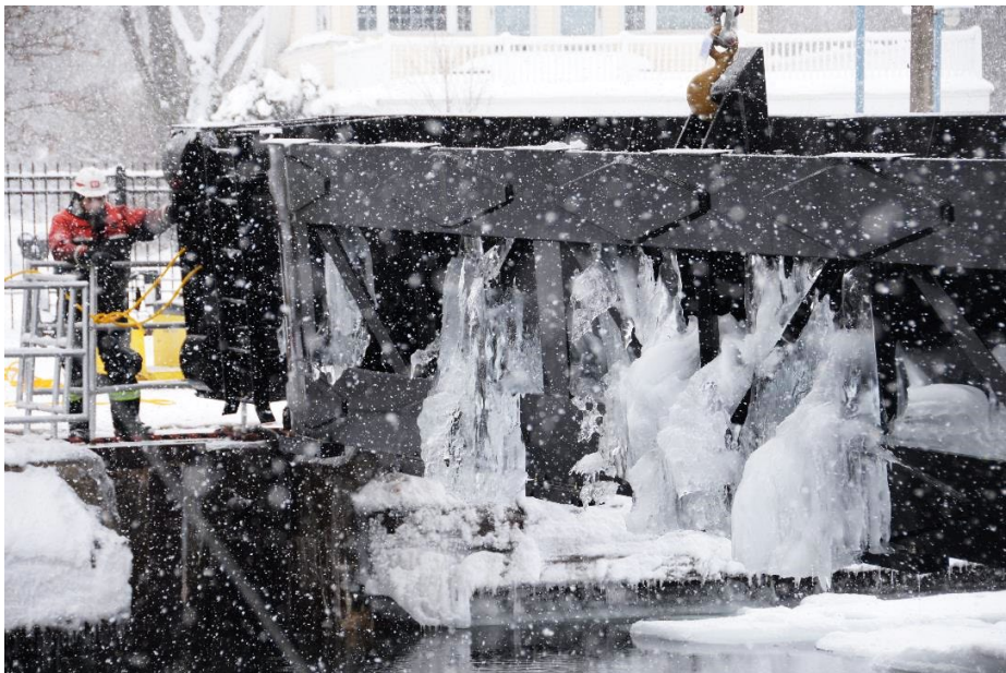
Removing a dewatering bulkhead
