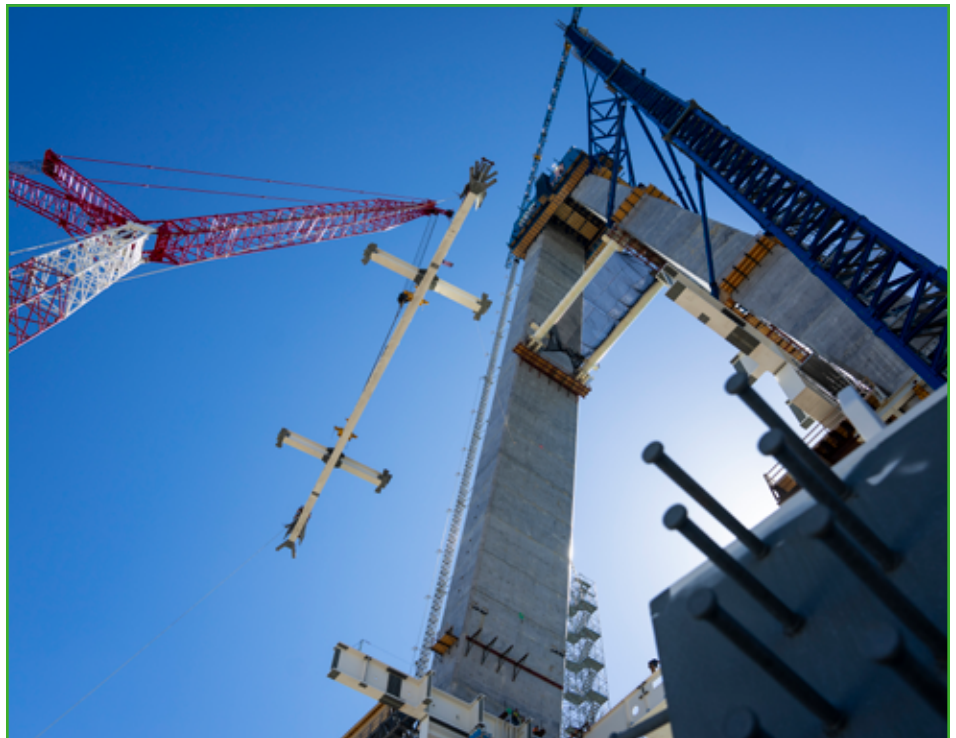
A crane is lifting a girder for the bridge road deck near the U.S. tower for the Gordie Howe International Bridge. (Photo courtesy of the Gordie Howe International Bridge project.)
