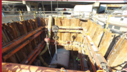
PRO-BRACE HYDRAULIC FRAME
