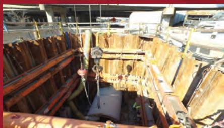
PRO-BRACE HYDRAULIC FRAME
