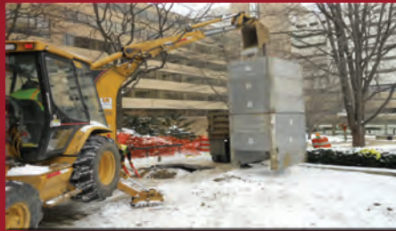
ALUMINUM TRENCH SHIELDS
