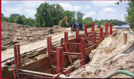
SLIDE RAIL SHORING
