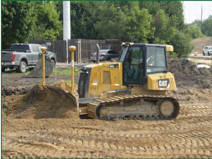
A CAT D6K2 LGP dozer pushes dirt on the U.S. 12/M-17 project in Ypsilanti Township.
