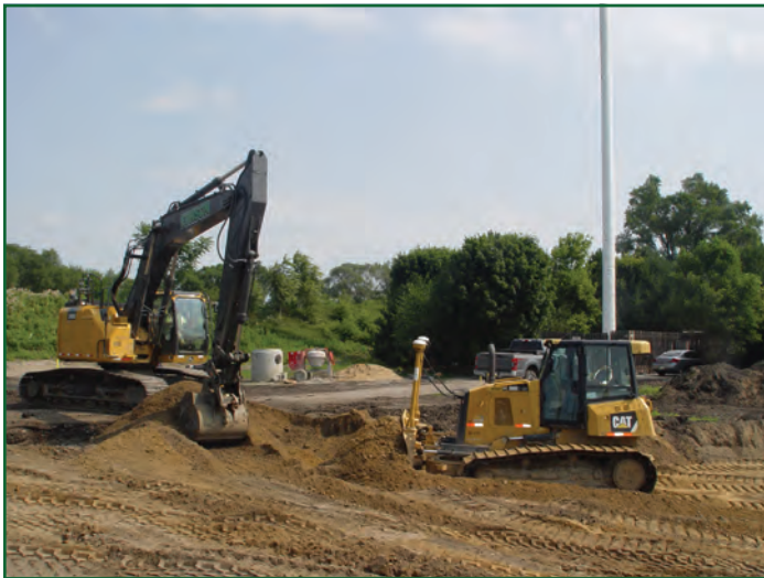
A CAT D6K2 LGP dozer and a John Deere 345G LC excavator work on the U.S. 12/M-17 project in Ypsilanti Township.
