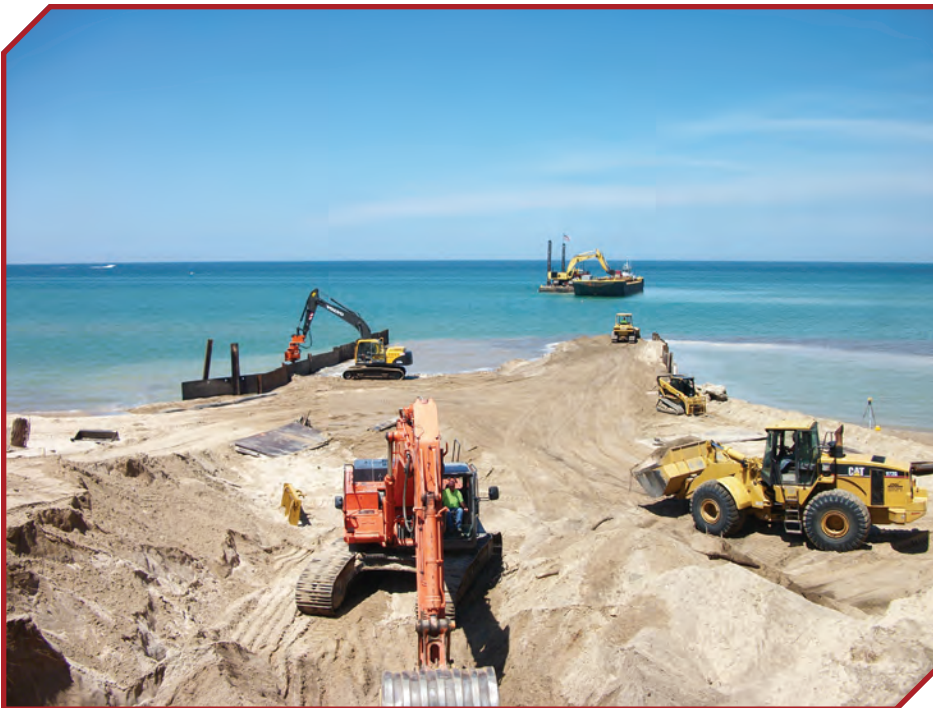
Constructing a temporary peninsula in Lake Michigan as part of a water intake construction project in Benton Township.
