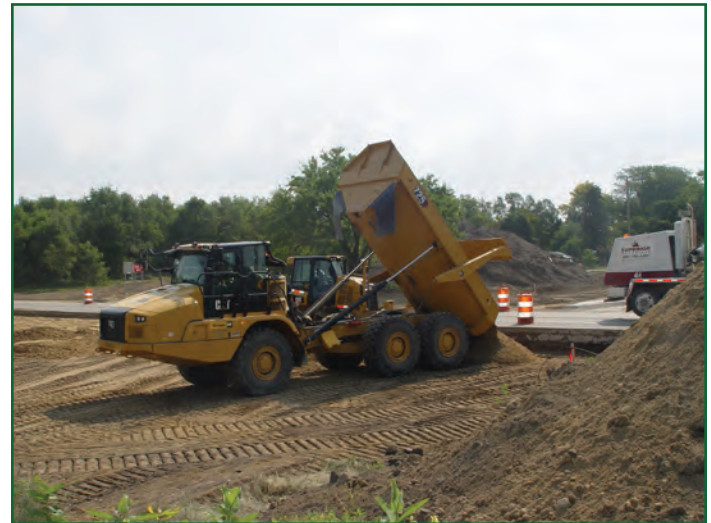
A CAT articulated truck unloads dirt on the U.S. 12/M-17 project.
